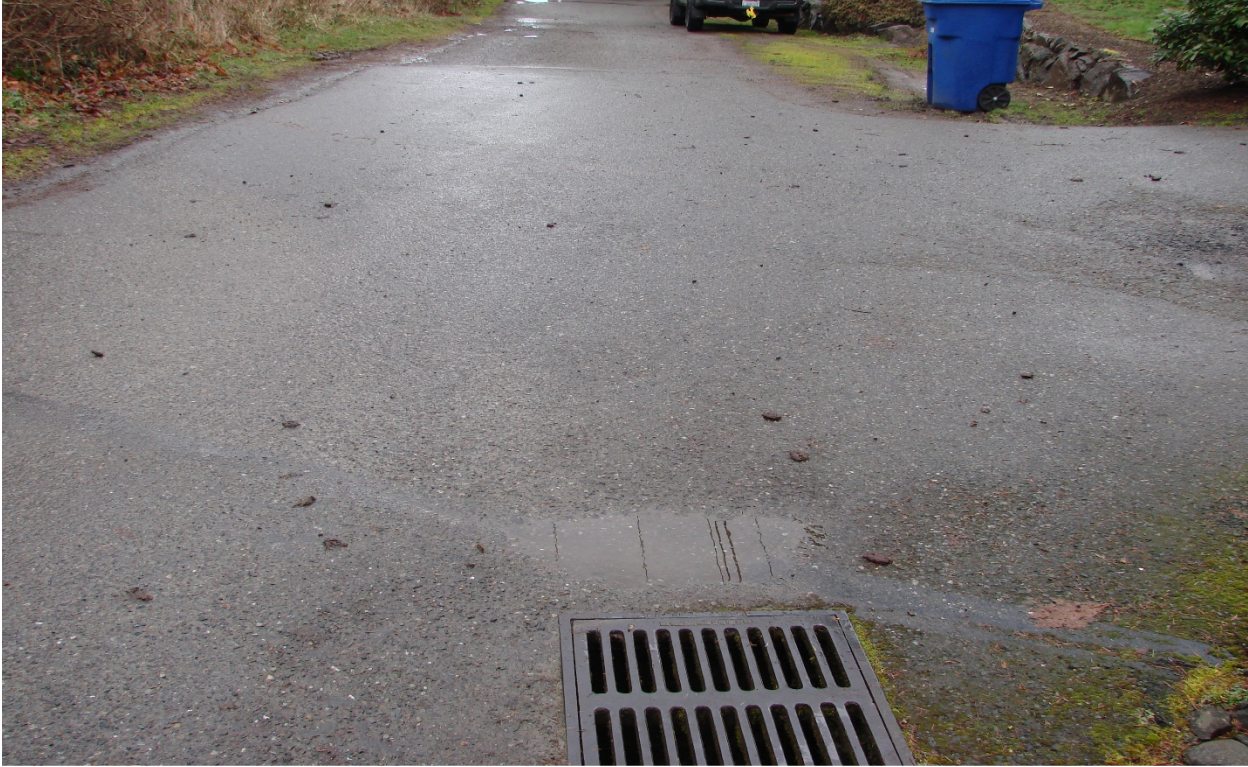
Photo #4 – Existing CB#28b-48 – viewing north on 80 th Avenue SE
