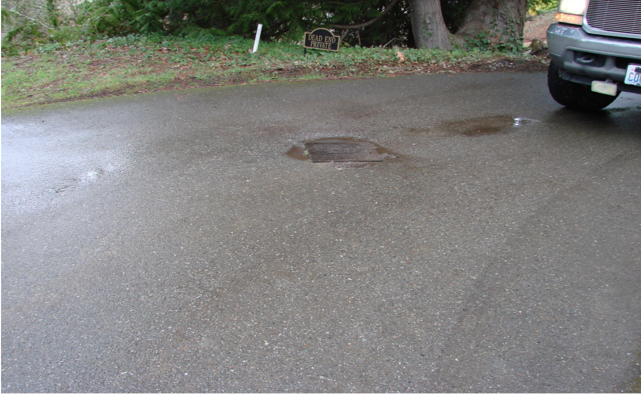
Photo #6 – Existing CB#28b-75 at end of 80 th Avenue SE
