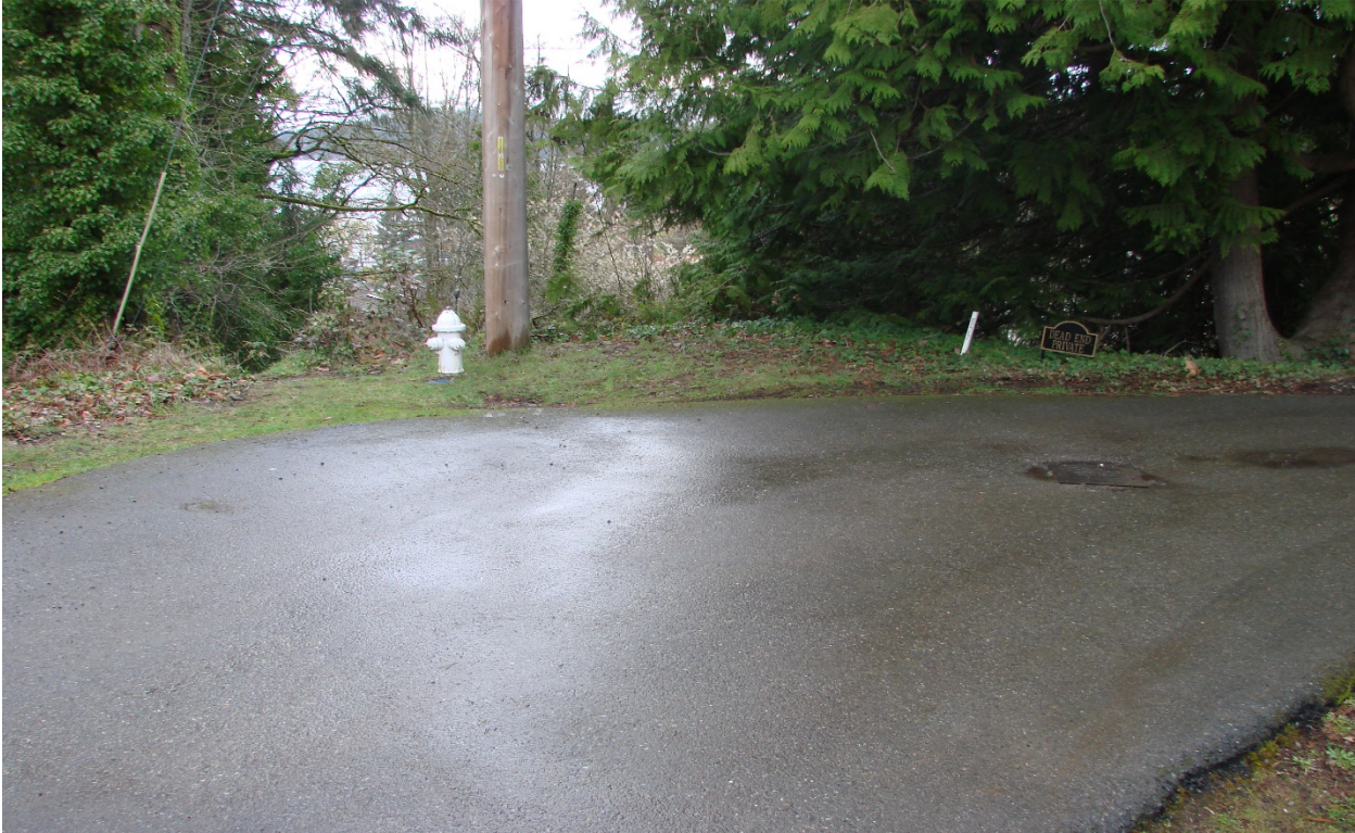
Photo #7 – North end of 80 th Avenue SE – before dropping down slope
