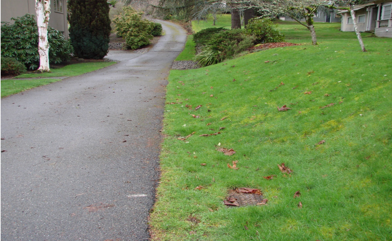
Photo #3 – Existing area drain on south side of driveway heading towards 8020 SE 57 th Street
