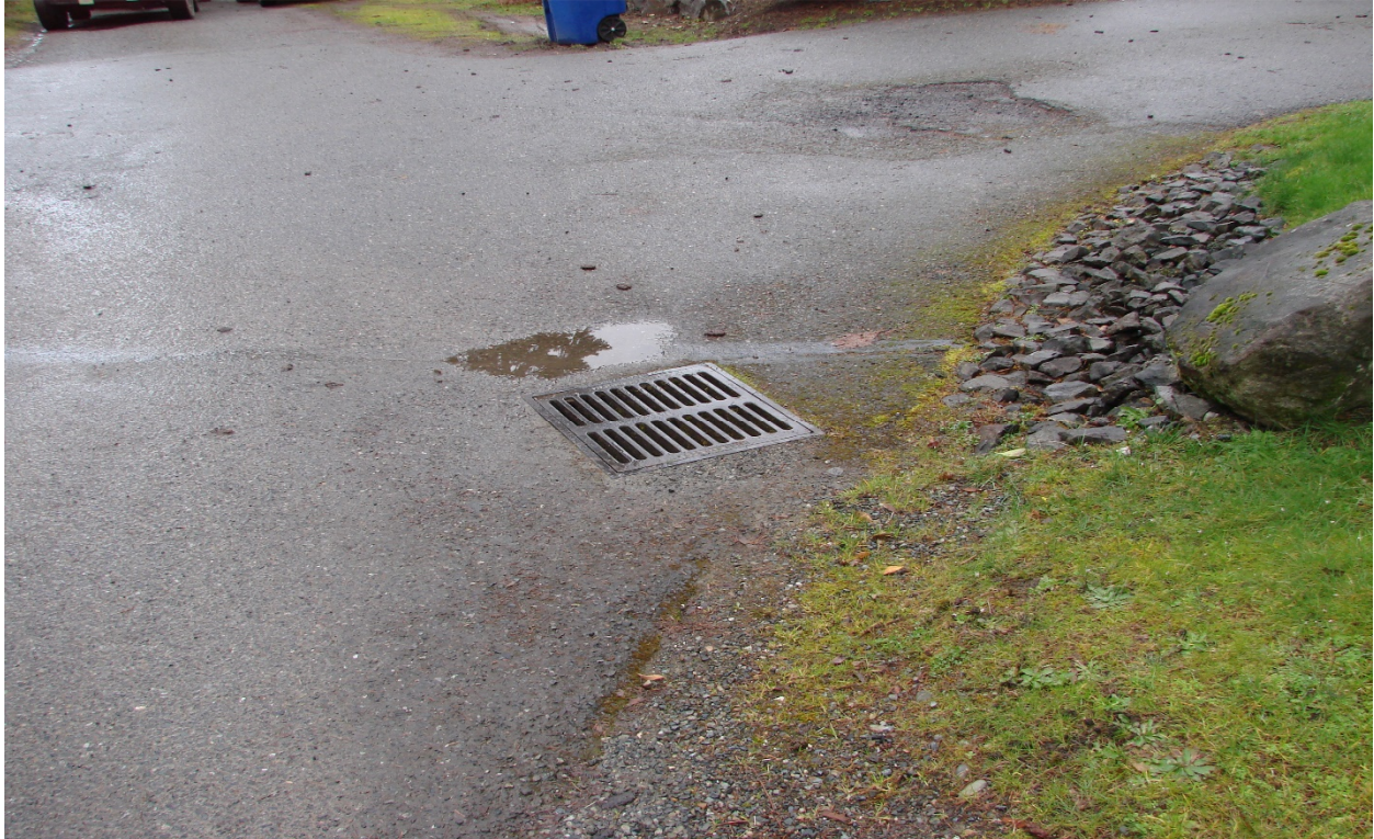
Photo #1 – Existing CB#28b-48 -within east side of 80 th Avenue SE
